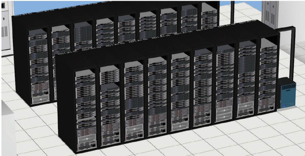
Figure 12. Example data center
